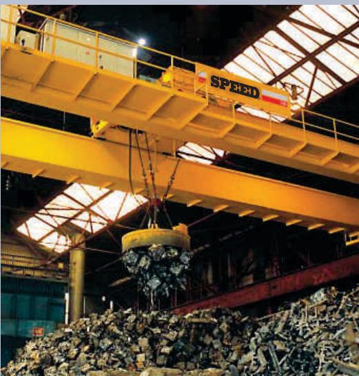
Scrap handling magnet crane
